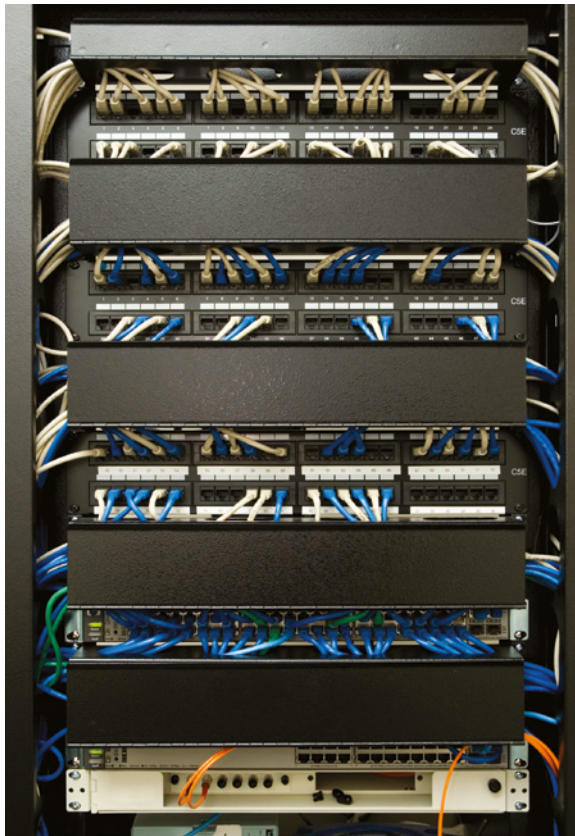
FIGURE 11.2 A wiring closet
