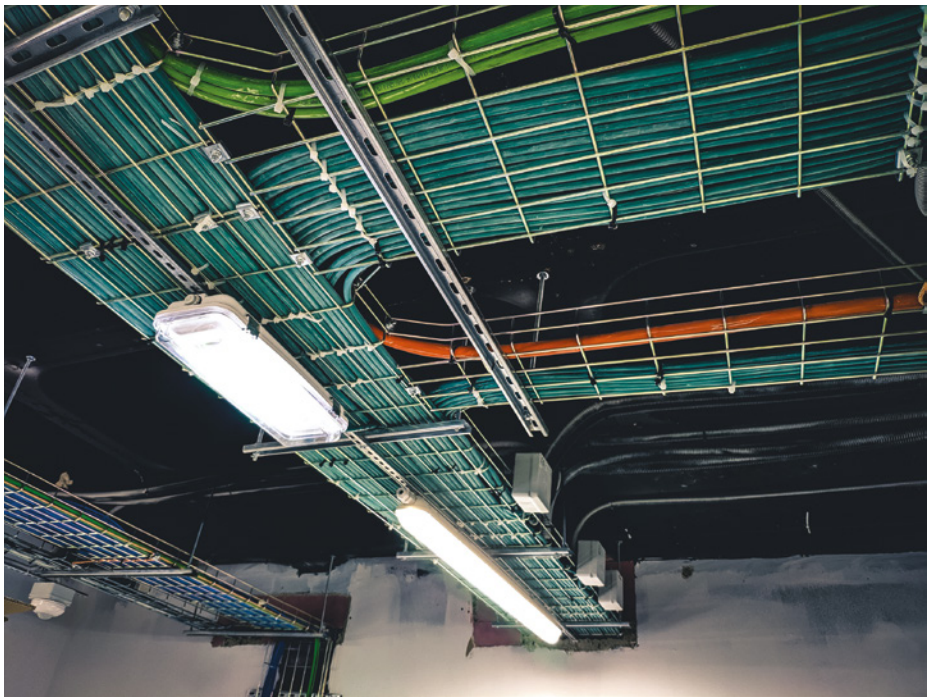
FIGURE 11.3 Cable distribution runs
