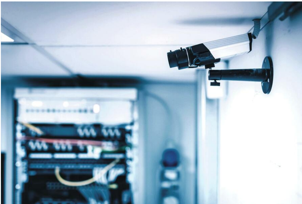
Pan-tilt-zoom CCTV installed to monitor a server room. (Image by Dario Lo Presti © 123RF.com.)
