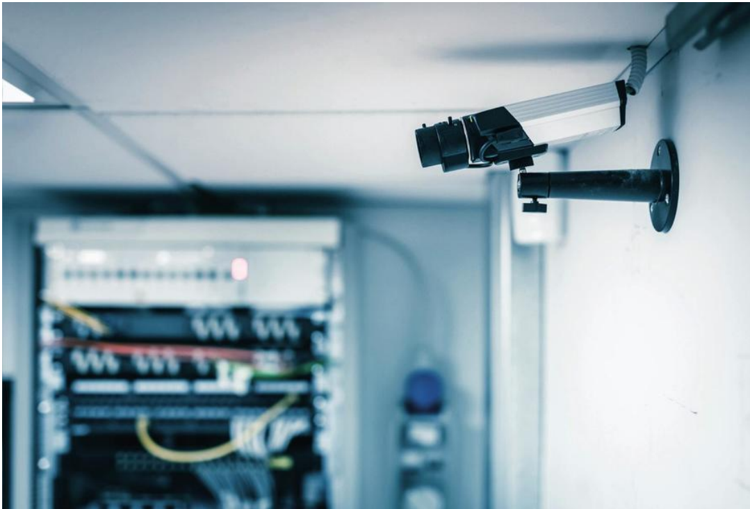
CCTV installed to monitor a server room. (Image by Dario Lo Presti © 123rf.com.)
